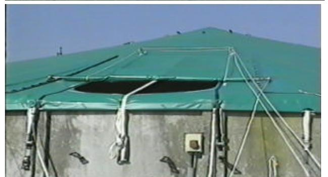
The Cover is resting on cords, these cords is fasten on the tank with a special developed hardware.
